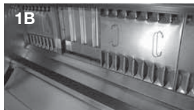
Grease-X-Tractor™ filters, first row of filters
