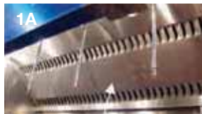
Grease-X-Tractor™ filters, first row of filters
